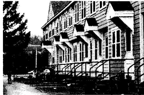
A $6.3 million energy efficiency and weatherization project is expected to trim energy costs at the Curwin Circle mixed housing development, above. Item photo / Reba M. Saldanha
